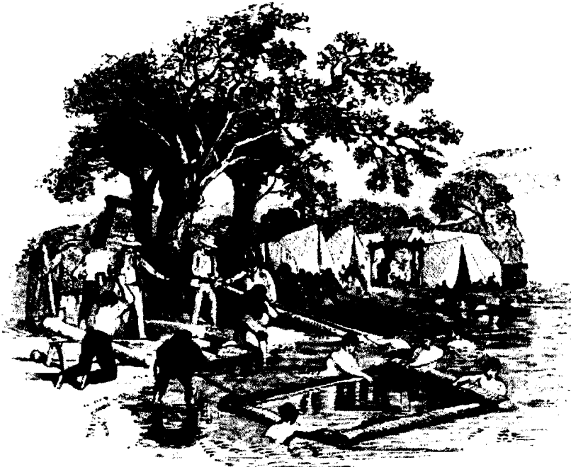
MORMONS BUILDING A BRIDGE.
